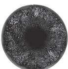
**Third stage** — a large amount of creosote/tar is encrusted on the pipe lining. It is highly recommended to hire professional at this stage.
